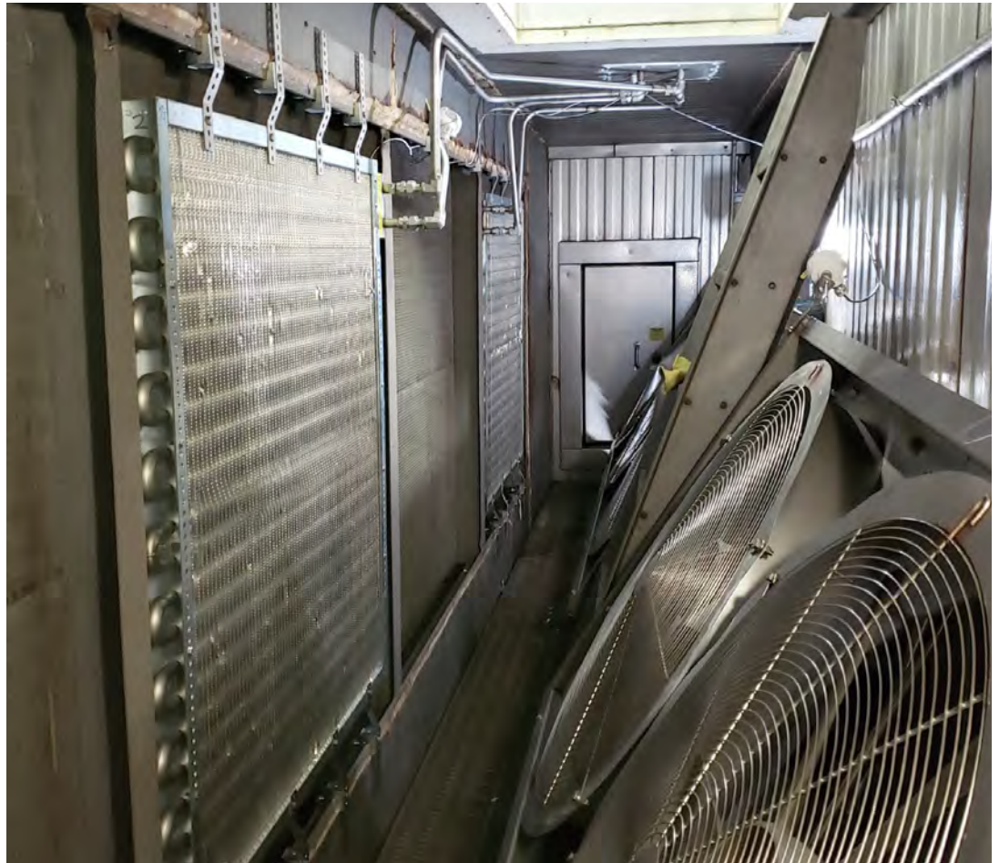
Example interior view of blast freezer equipped with NITROBOOST BL system.
